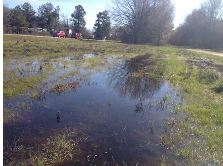
Photo 14: Wetland within project area on south side of current US-82 alignment.
