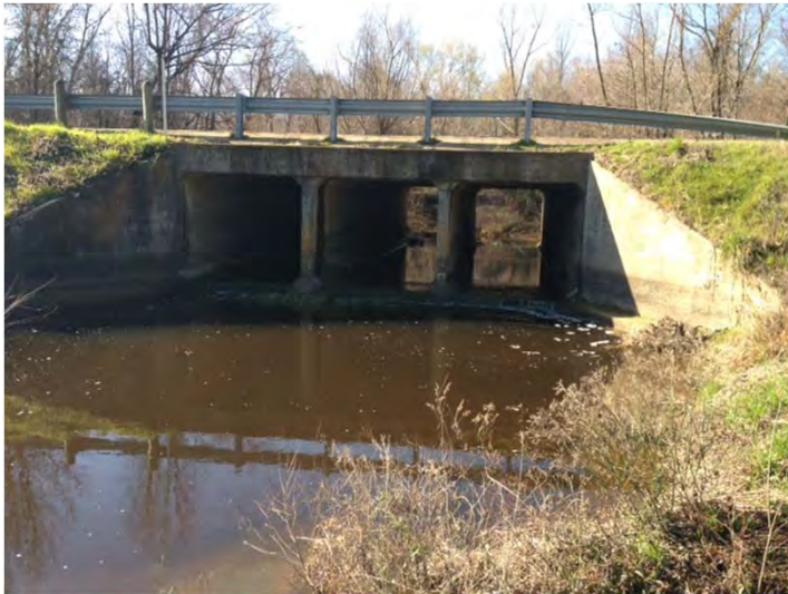
Photo 9: North side of box culvert over Red Bayou.
