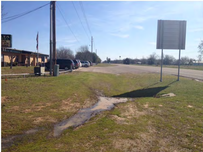
Photo 15: View of north side of current US-82 right of way, adjacent to Malta School.
