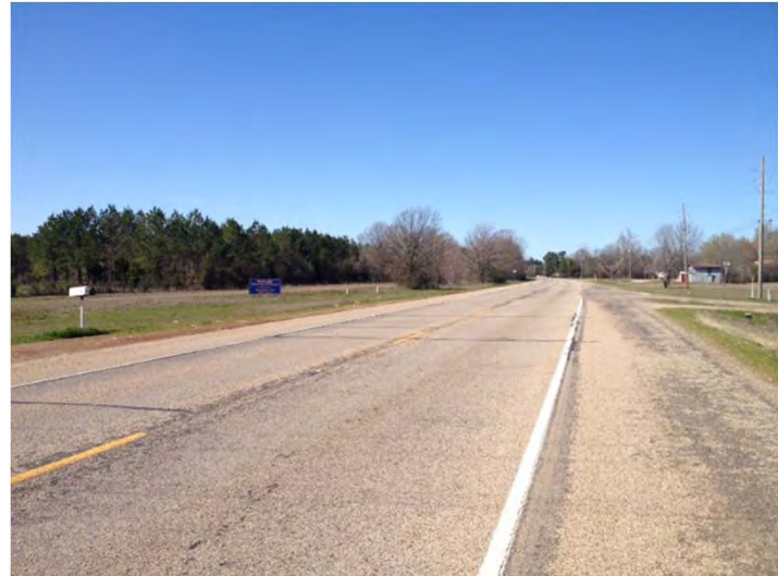
Photo 20: View of project area near western extent of corridor; view to northwest.
