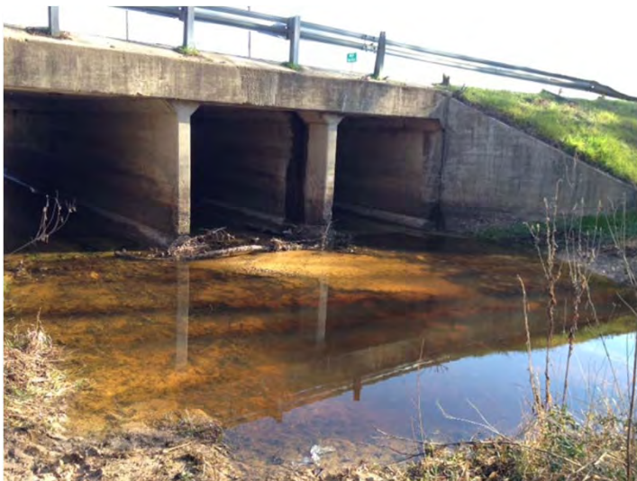
Photo 11: South side of box culvert over Red Bayou.
