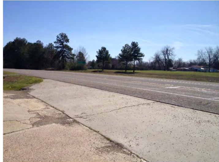
Photo 22: View of typical vegetation within and adjacent to US-82 and railbank.
